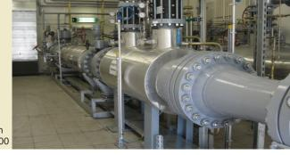
Horizontal Preheater: Flow rate: 80.000m<sup>3</sup>n/h Design pressure: PN100
