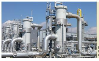
Filter-Separator: Flow rate:491.000 m<sup>3</sup>n/h Design pressure: 84 bar
