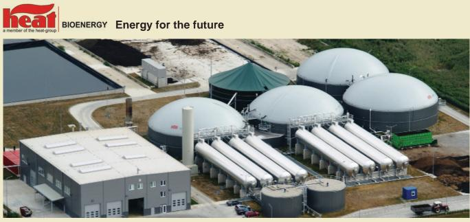
The biogas plant BOSANY is located 50km from Nitra (Slovakia). HEAT Bioenergy as a general contractor designed and built the complete plant on turn-key basis. The plant, which started its opertions in 2012, is designed to process approx. 100.000 t/y of organic residues and renewables, with an electric generation capacity of  $2 \times 1.4$  MW.
